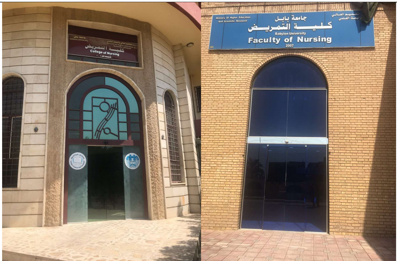
Setting the main doors with sensors to be closed and opened in need only to reduce the energy of air-conditioning.
